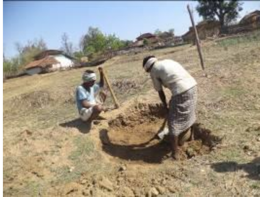
Bhagpur- Compost pit built with our assistance at Indram Maravi's house
