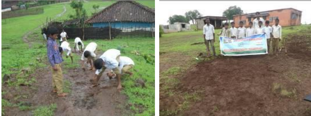
Batwar- School road site before (left) and after (right) our programme
