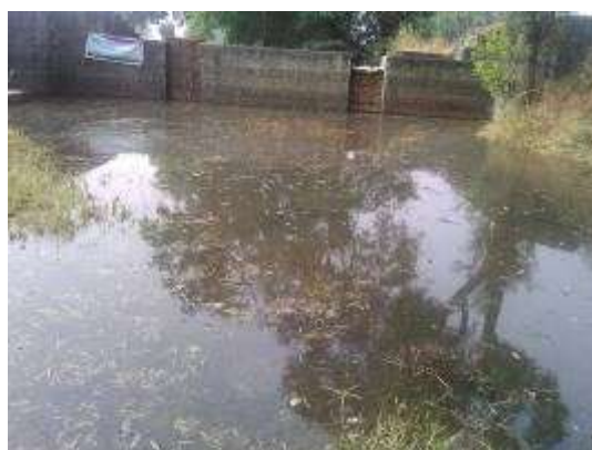
Check dam built by our team
