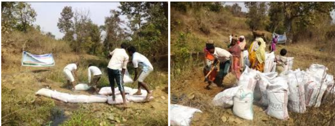
Volunteers build dam using locally available materials
