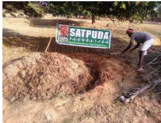
Manegaon - Compost pit built with our assistance at Hironidibai Markam's house
