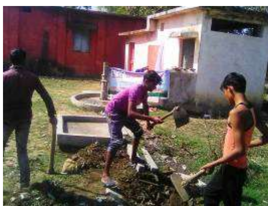
Volunteers clear area around hand pump and dig a fresh soak pit
