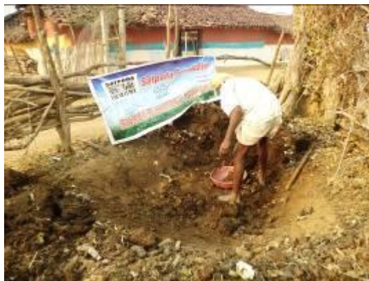
Manegaon- Compost pit built with our assistance at Sukhman Dhurwey's house
