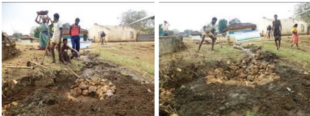
Volunteers clear area around hand pump and dig a soak pit
