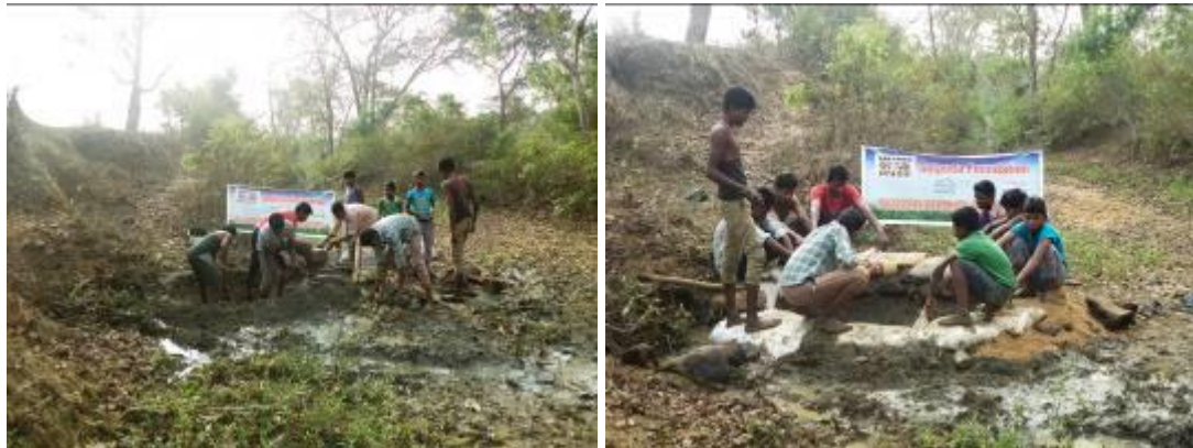
Volunteers build water tank using locally available materials
