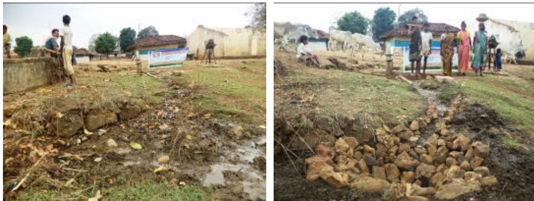
Batwar- Hand pump site before (left) and after (right) our programme
