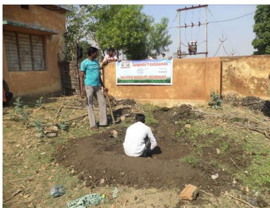
Patpara- Compost pit built with our assistance at Sanokhi Bai's house
