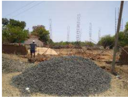
Patpara - Construction of "Rangmanch" commenced as per the micro-plan
