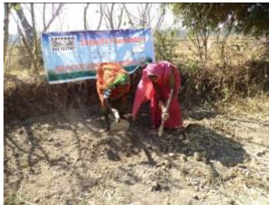
Manegaon - Compost pit built with our assistance at Kasturi Bai's house
