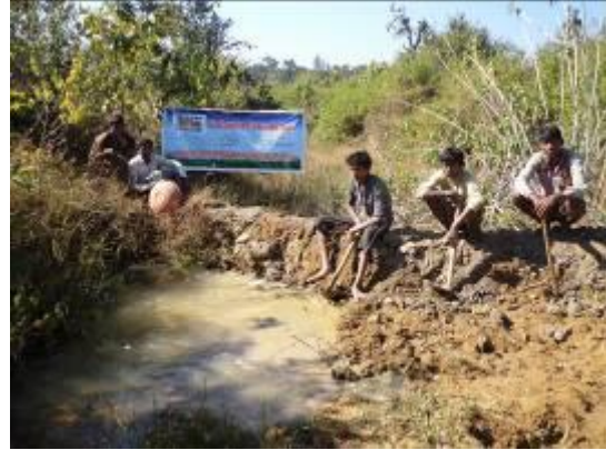
Volunteers poses after check dam is built
