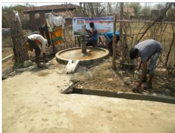
Volunteers clean area around hand pump at Asalpani
