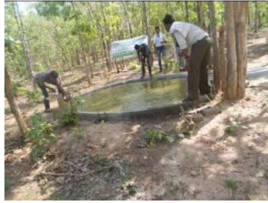
Cleaning water hole in Comp. no. 108
