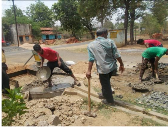
Volunteers clean area around hand pump at Bodalkasa and dig soak pit
