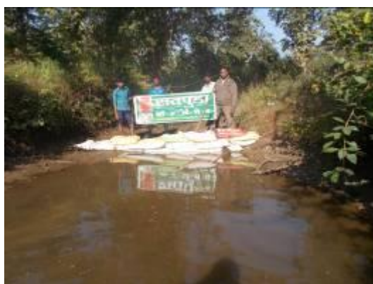
Check dam built in Compartment no. 56
