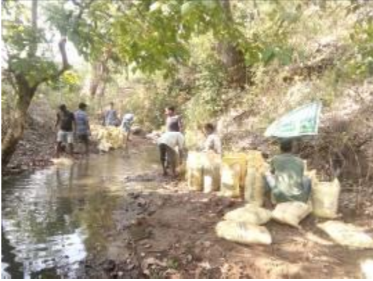
Khapa - Dilip leads villagers in building check dam
