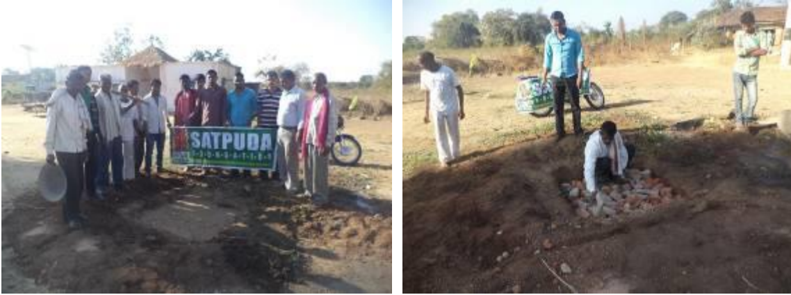
Team digs soak pit at Ghoti village
