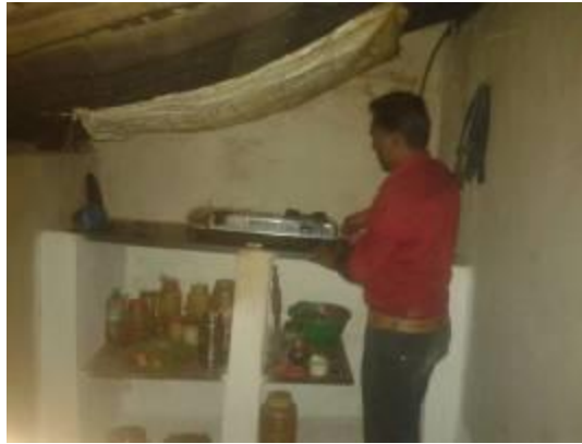
Niranjan repairing biogas stove in Aamajhiri village
