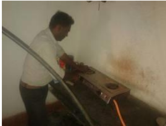
Niranjan repairing biogas stove unit in Aamajhiri village
