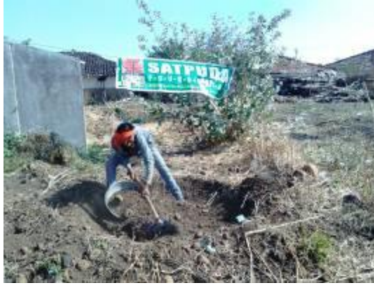
Mohgaon - Compost pit built with our assistance at Rajkumar Bhalerao's house
