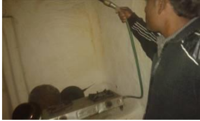
Niranjana repairing a biogas unit in Aamajhiri village
