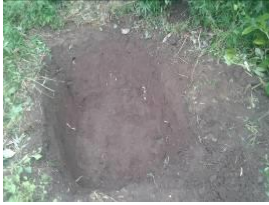
Aamajhari – Villagers prepare compost pit
