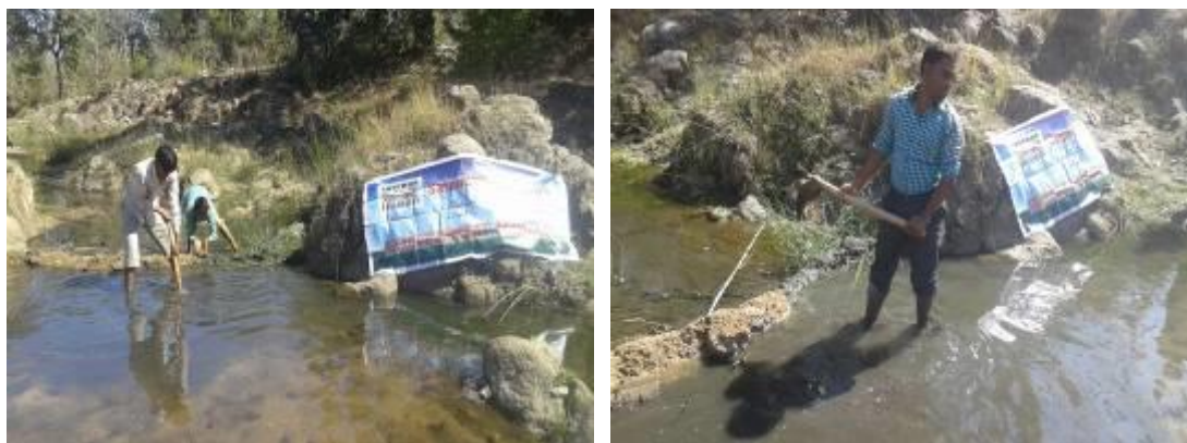
Team builds check dam near Khamba village
