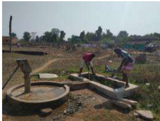
Durgapur – De-silting of percolation tank next to a hand pump
