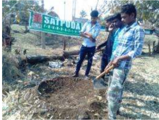
Chirrewani – Volunteers construct compost pit
