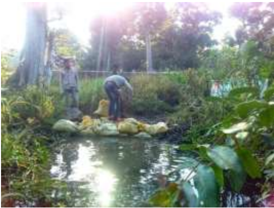
Construction of check dam near Mohgaon village by volunteers
