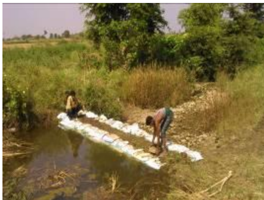
Villagers constructing check dam on a stream near Kundai village
