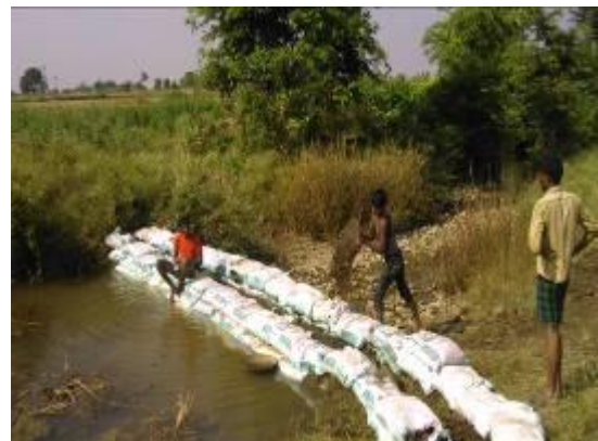
Villagers constructing check dam on a stream near Kundai village
