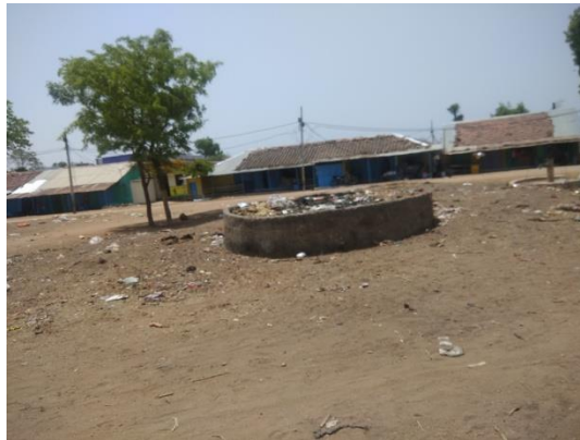
Solid waste management tank at Matkuli market area
