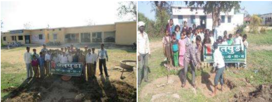
Soak pit dug at GPS Pisuwa (left) and GMS Pisuwa (right)
