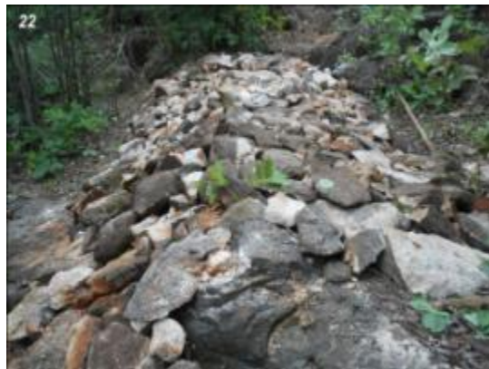
Jhirpa – Check dam being built
