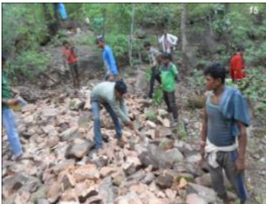
Jhirpa – Check dam being built
