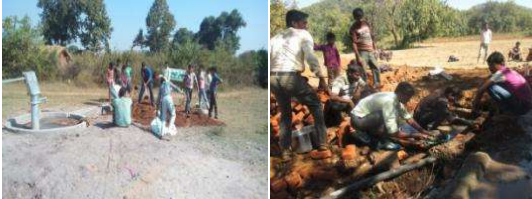
Soak pit dug at Matkuli (left) and Bindakheda (right)
