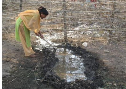
Mudholi - Cleaning of area around hand pump
