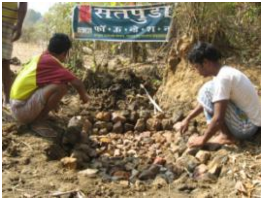
Udiya Tola – Team digs canal to take spill over water from hand pump to water hole
