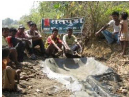
Water hole built at Udiya Tola in programme organised by us
