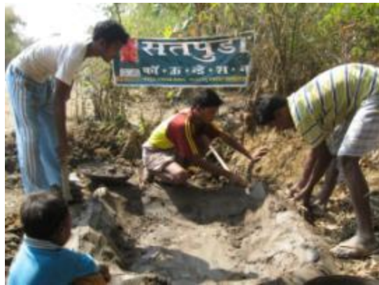
Udiya Tola – Team digs canal to take spill over water from hand pump to water hole
