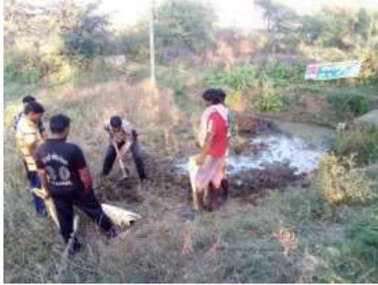
Mudholi – Villagers construct a check dam through shramdhaan
