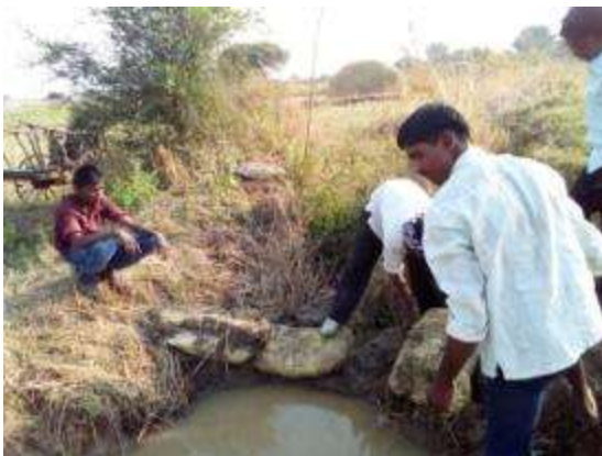
Khutwanda - Villagers construct a check dam
