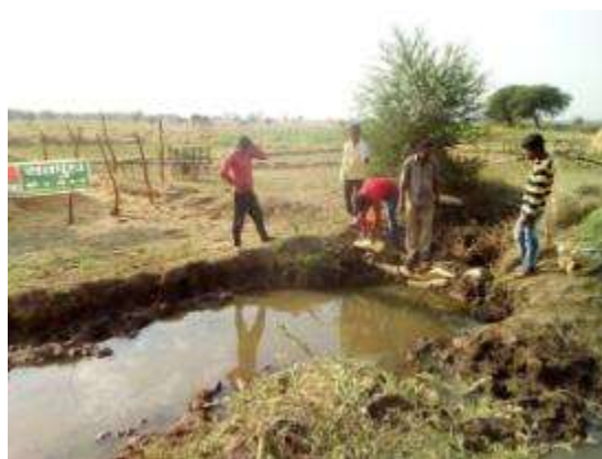
Mudholi - Villagers volunteer to construct a check dam
