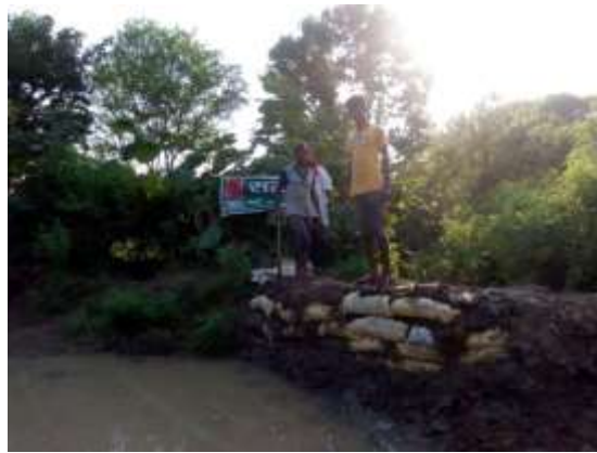
Mudholi: Check dam completed
