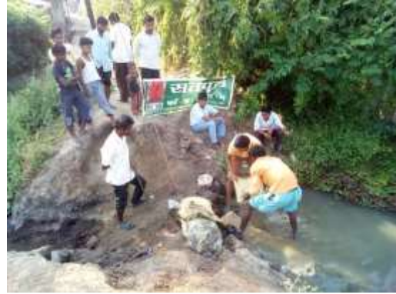
(Left) Villagers construct check dam at Mudholi and (right) at Junona
