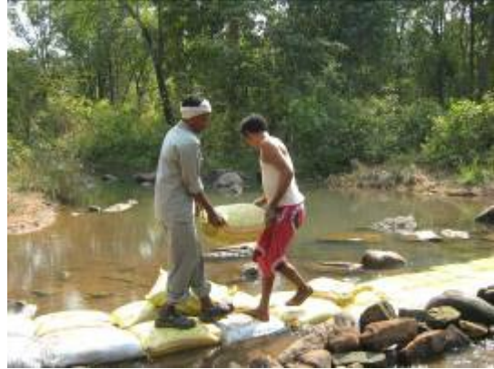
Check dam being built at Anjandana
