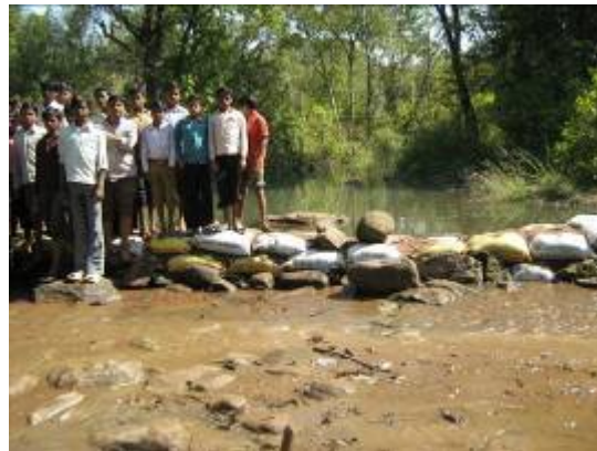
Check dam being built at Nayakheda
