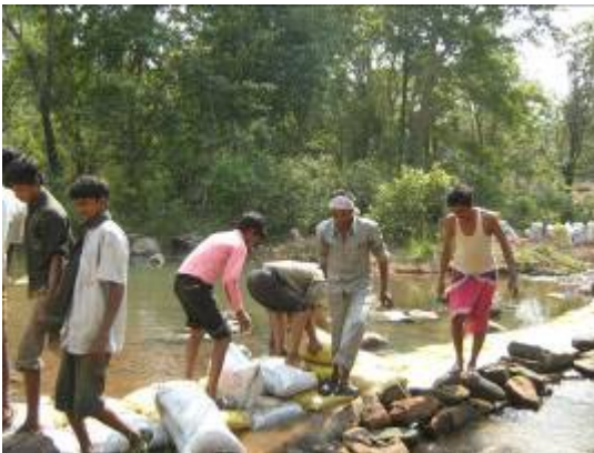
Check dam being built at Nayakheda
