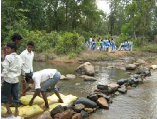
Check dam being built at Anjandana
