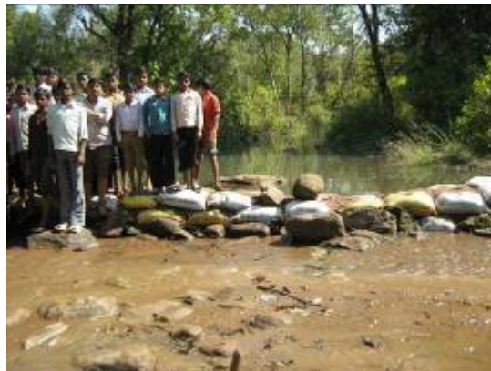
Check dam being built at Nayakheda
