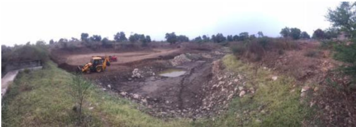
Panoramic view of the recharge lake in Telgaon
