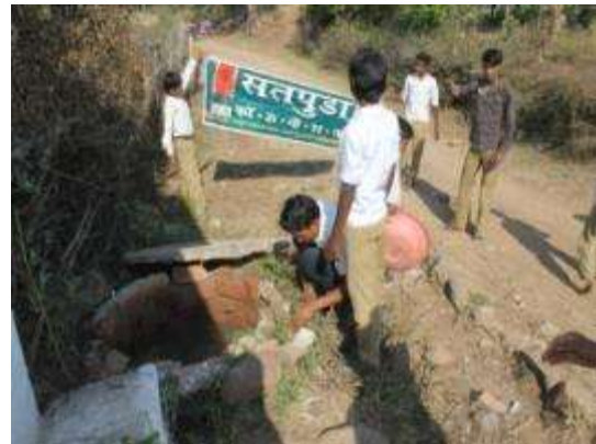
Digging soak pit at Jhirpa (left) and Matkuli (right)
