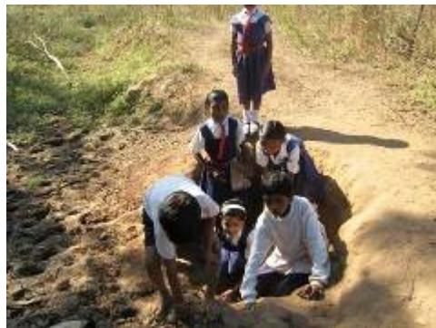
Students of ZP School, Adegaon (Tadoba) dig soak pit to take spillover water from hand pump
