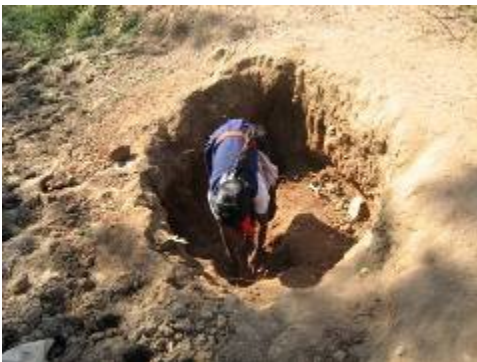
Students of ZP School, Adegaon (Tadoba) dig soak pit to take spillover water from hand pump
