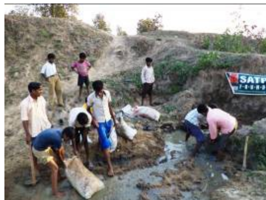
Check dam being built at Bawanjodi nala at Chapri
