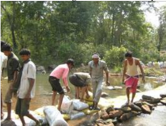
Check dam being built at Anjandana, Satpura Tiger Reserve
