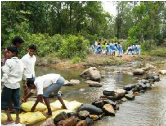
Check dam being built at Satdhara, Anjandana
