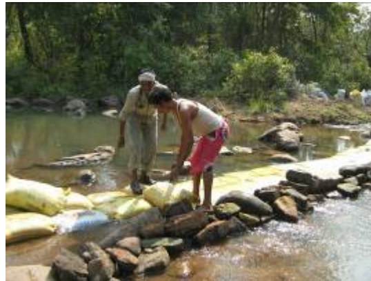
Check dam being built at Anjandana, Satpura Tiger Reserve
