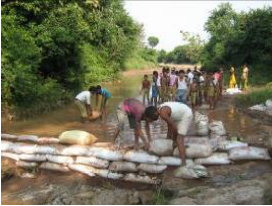
Programme to build stop dam at Bindakheda nallah, Matkuli
