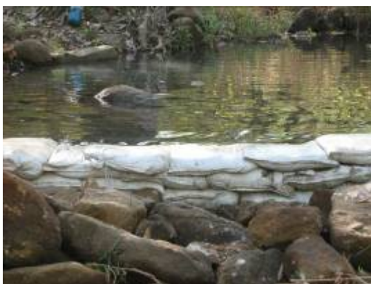
Stop dam at first site at Raikheda
