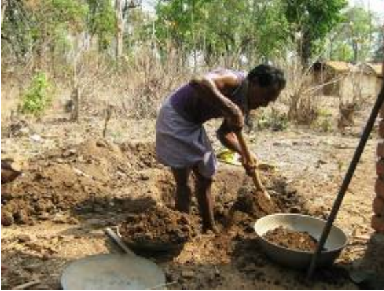
Soak pit being dug at Kondegaon
