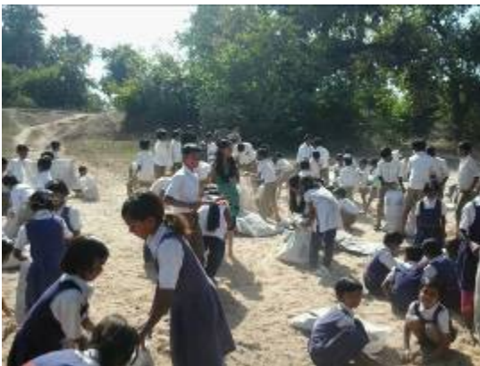
Aamajhari - Students filling bags with sand to use in building check dam
