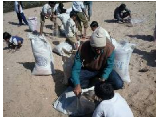
Aamajhari - Students filling bags with sand to use in building check dam
