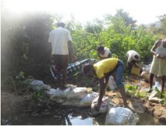
Khapa -Check dam being built
