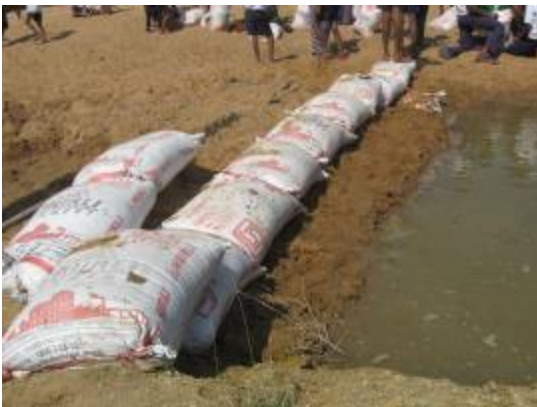
Chorgaon - Check dam being built
